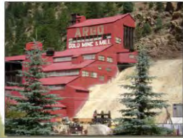
7. View north to Argo Gold Mine
