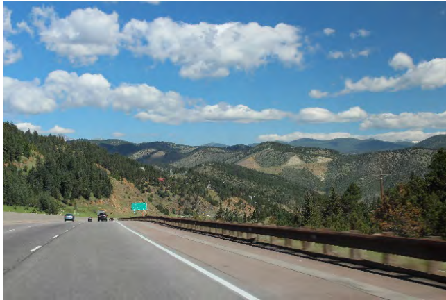
Exhibit C6. View 5 - Northbound view from I-70 near Milepost 247 (LU-1)
