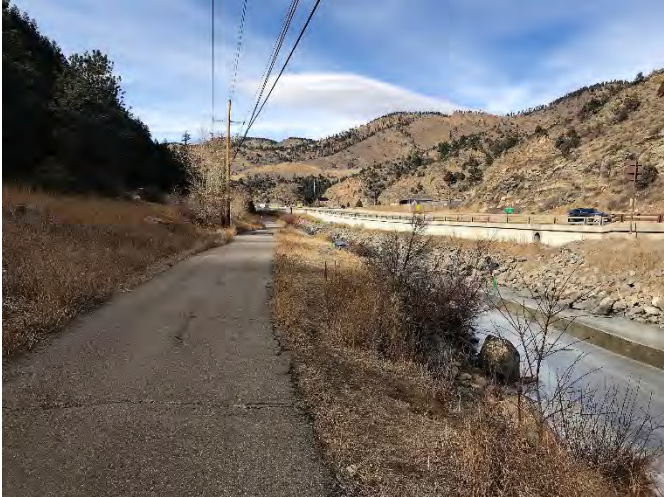
Exhibit C24. View 24 - Westbound view from Greenway, Clear Creek and I-70 (LU-3)
