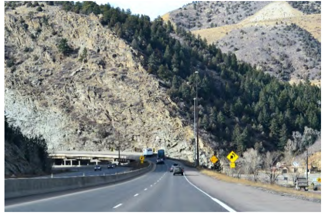
Exhibit C12. View 11 - Westbound view of US 6 offramp (new tunnel approach) (LU-2)
