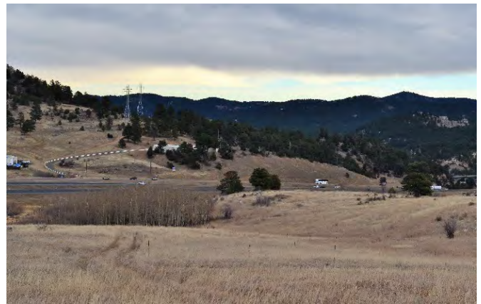
Exhibit C5. View 4 - Eastward view of wildlife crossing from the Clear Creek High School parking lot (LU-1)
