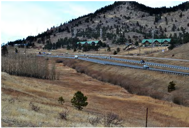
Exhibit C2. View 1 - West view of I-70 from Evergreen Lane north of Beaver Brook /Floyd Hill interchange (LU-1)
