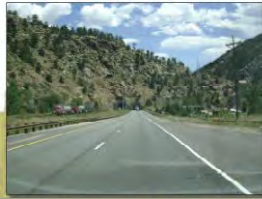
6. View east towards Idaho Springs
