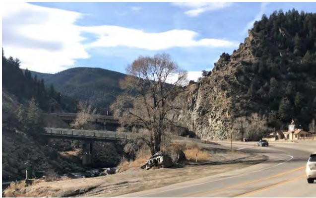
Exhibit C14. View 13 - Southbound view of US 6 offramp towards I-70 from in front of Quarry on US 6 (LU-2)
