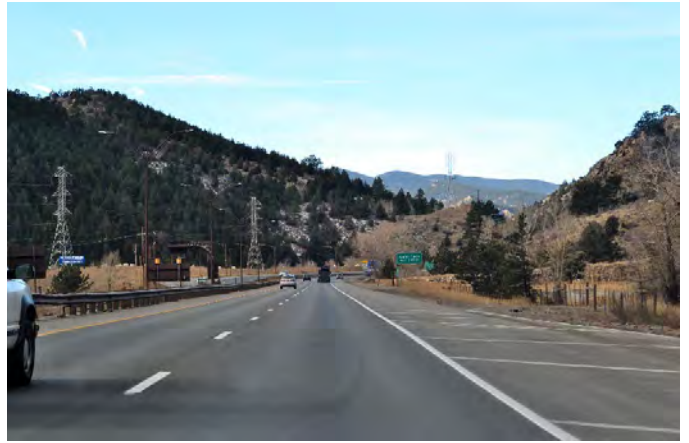
Exhibit C19. View 18 - Westbound view just west of Veterans Memorial Tunnels (LU-3)
